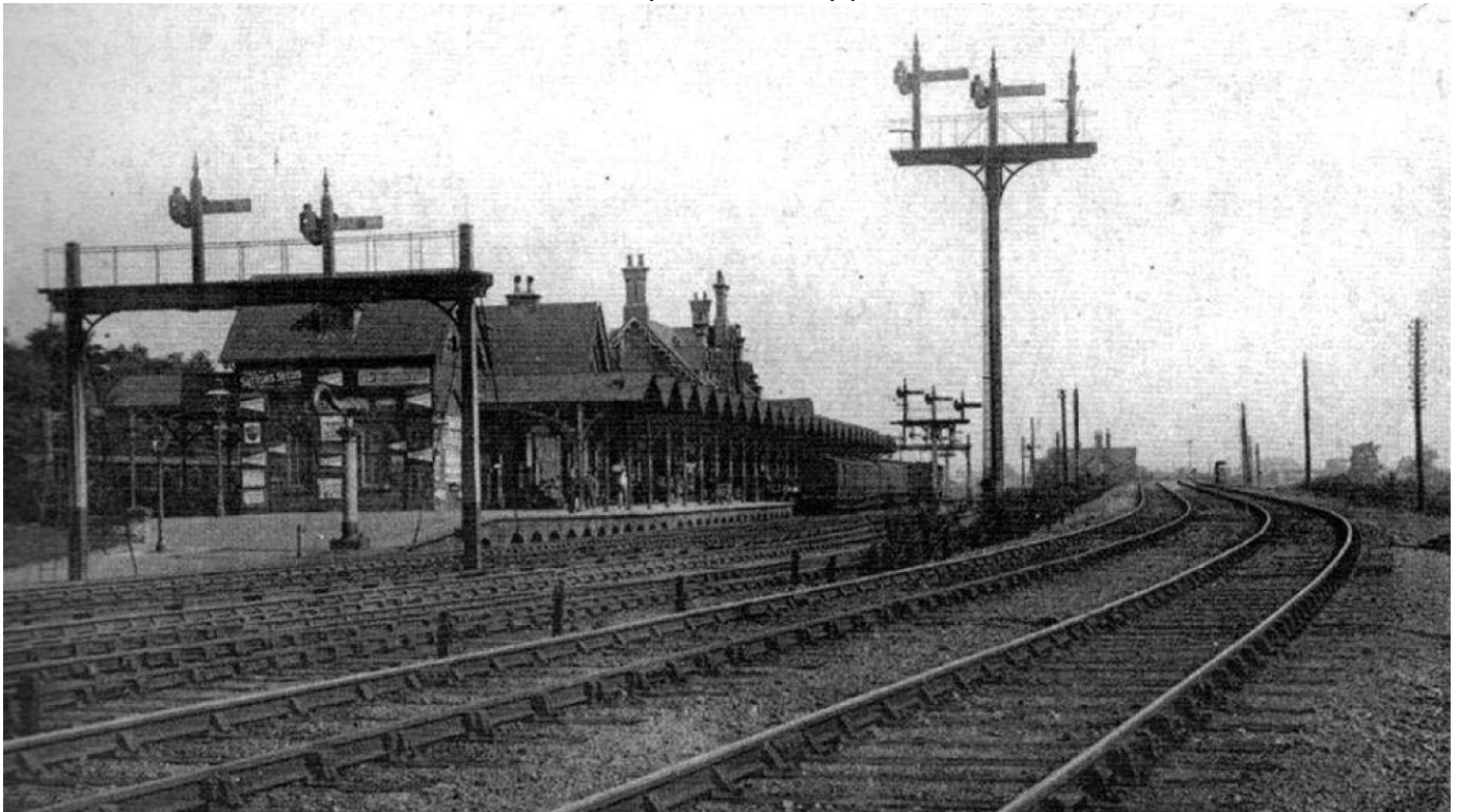
The goods line starts to rise to a higher level and moves away from the other lines as it passes Trent Station on its way to Toton marshalling yard.
